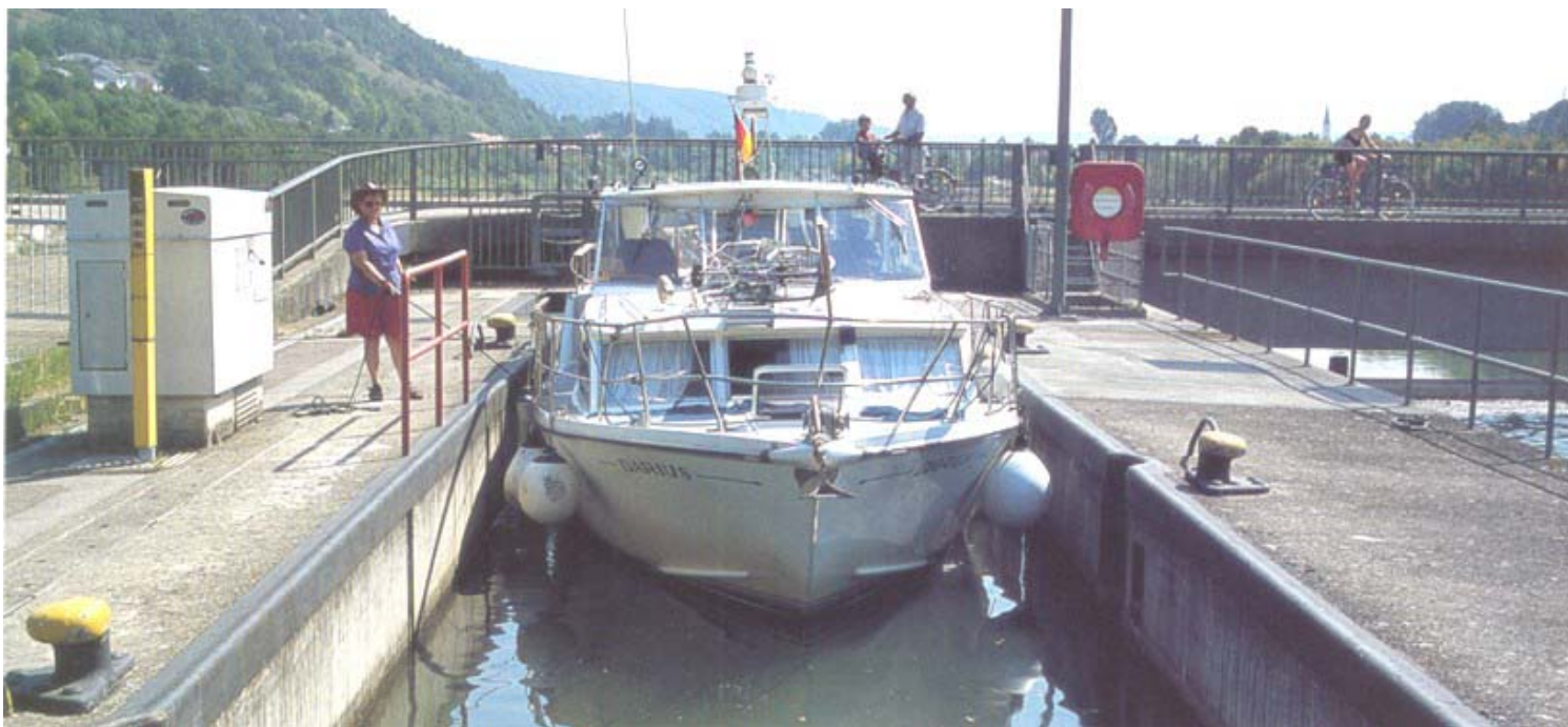
Darius at Kelheim lock, one of several on the Rhine-Main_Danube route, that has a small separate chamber to offer leisure craft a quicker passage.
